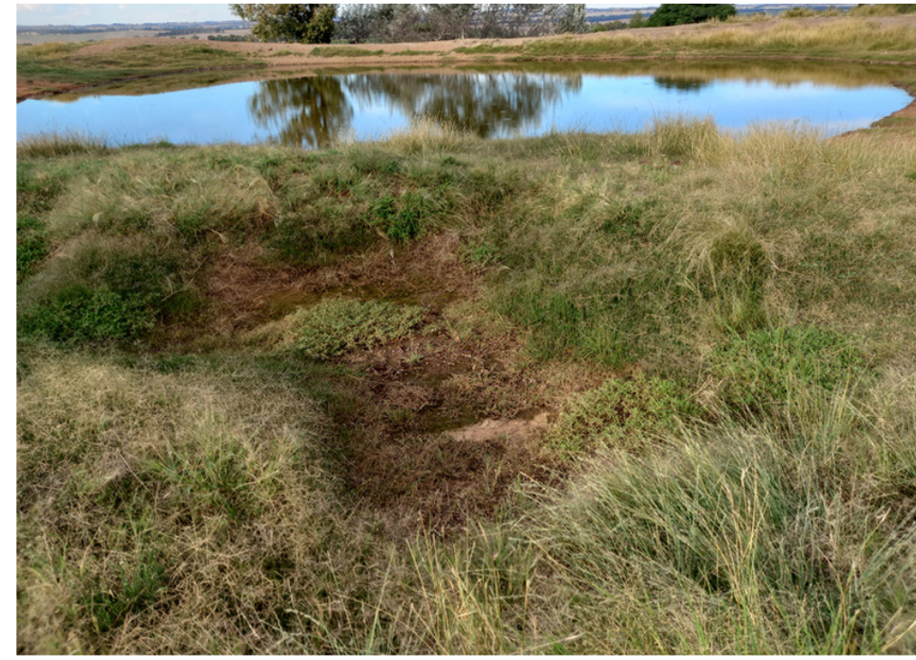
Figure 1: Dams constructed with silt-traps.
